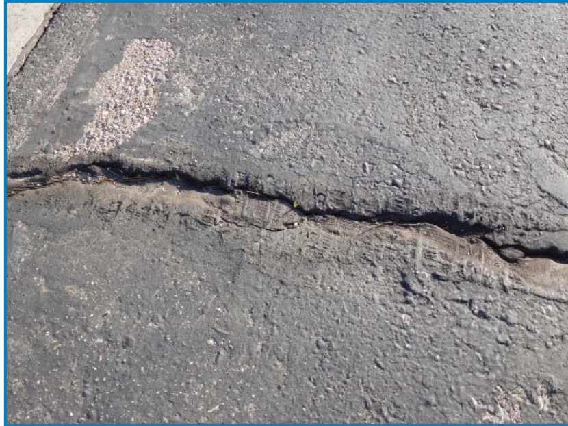
Asphalt cracking
